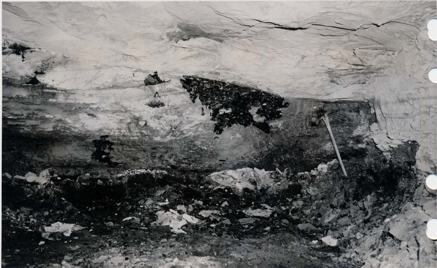
(5) North-west corner of west end of 12 main west. About 1' west of sta. 2575. Showing angular uncon- formity of siltstone over eroded coal. (6-10-56) Crown mine, Farmersville, Ill
