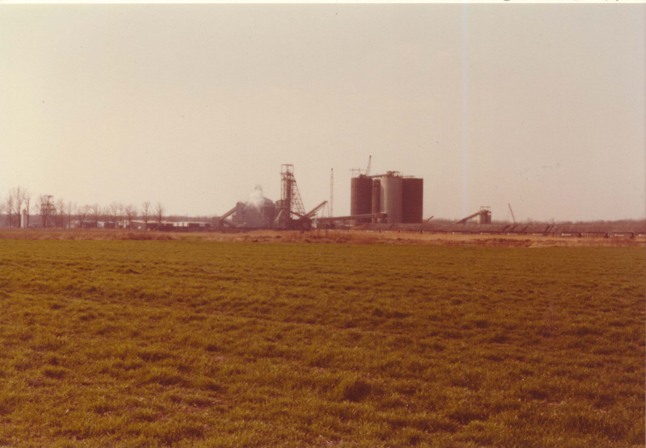
Surface works of Inland Steel Co. Mine No. 1, Jefferson County; as viewed from southeast. Photo by John Nelson, March 1981.
