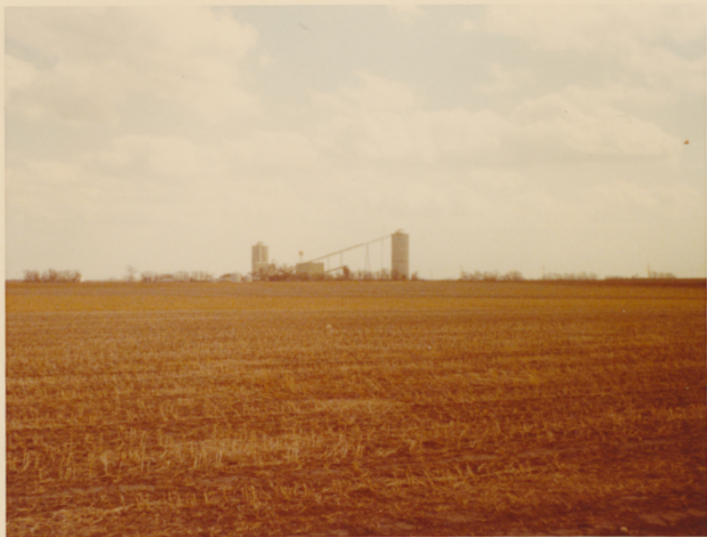
Tippel of Crown II Mine viewed from the northwest. This and the following color prints were taken by John Nelson in June 1976.
