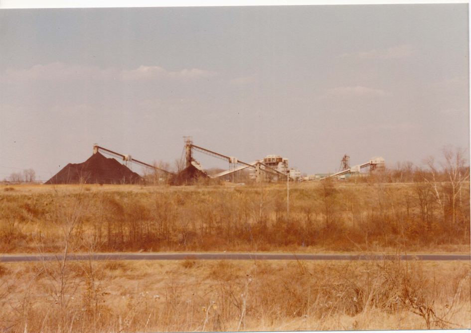
Surface works of Old Ben No. 26. Photo by John Nelson, March, 1981.
