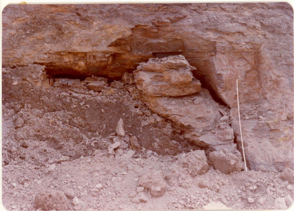
Another collapsed mine opening in the highwall. This fall has domed out in the Energy Shale, a gray, silty, sideritic shale. Ruler is 6 feet long.
