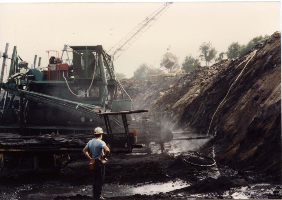
Overburden drill, Pit 3. Shot holes are drilled horizontally about 90 feet into the face, just above the coal bed.
