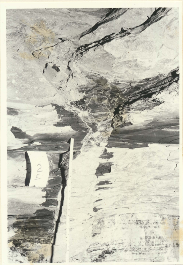
Same clay dike as in previous photo, opposite side of roof fall. Dike divides into thin fissures about 15" above the top of the coal bed, and bedding planes near the top of the coal are bent downward slightly.
