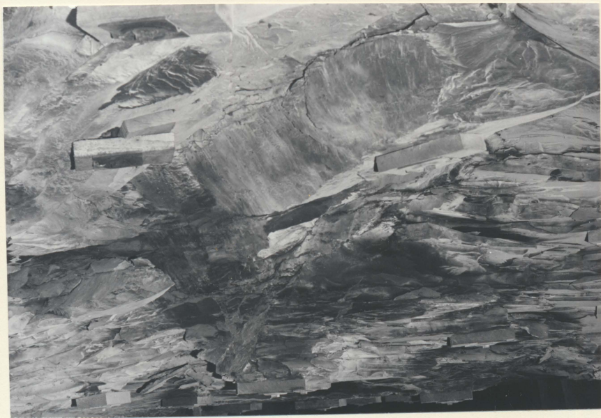
Different view of slip fracture along clay dike. This slip caused a roof fall here.
