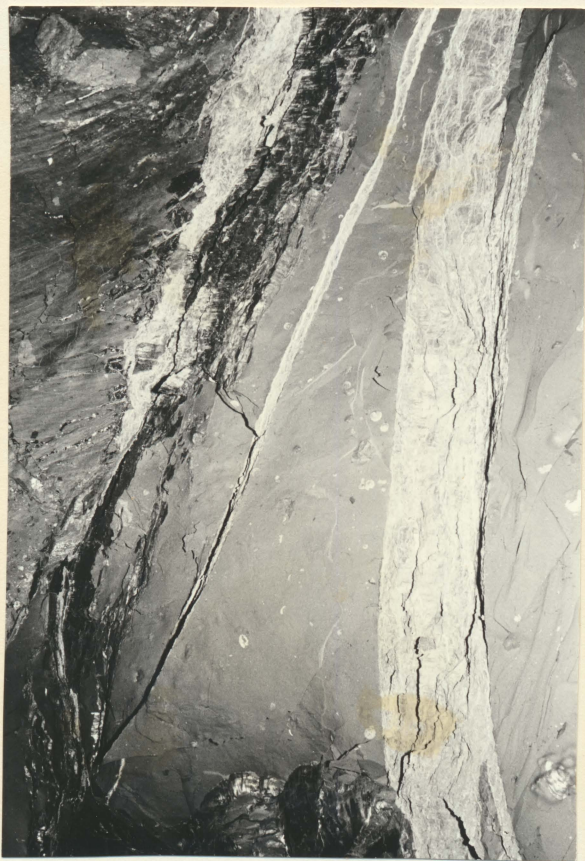
Trace of another clay dike (white) across the black shale of the roof.
