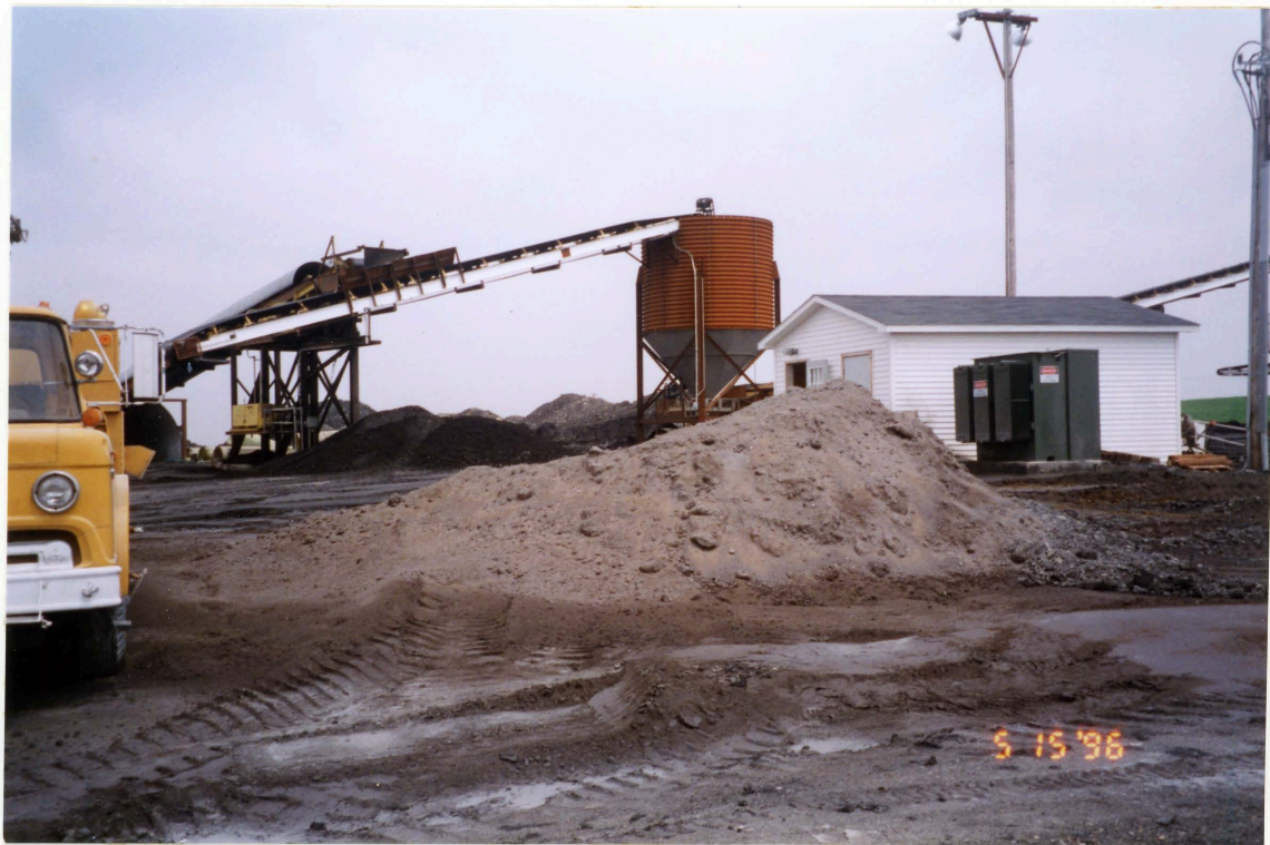
Conveyor belt from slope, Riola Mine
