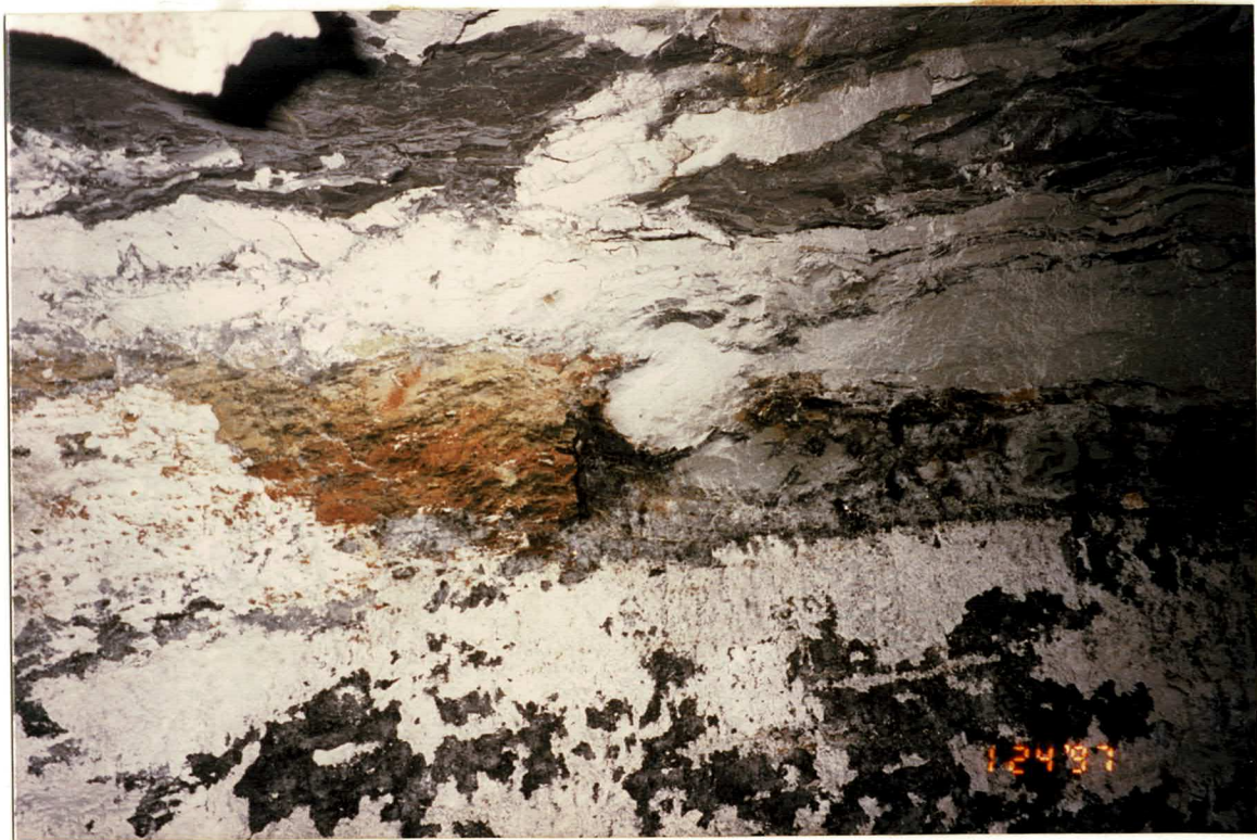
This photo was taken at location 3 or 4. Note disturbed roof sediments, micro faulting, sandstone veins, and irregular contact between coal and roof.
