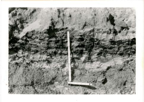
Stringers of coal and carbonaceous shale interbedded with soft clay and sand in North Side Mine. Apparently this is channel-fill material in Anvil Rock Sandstone interval.
