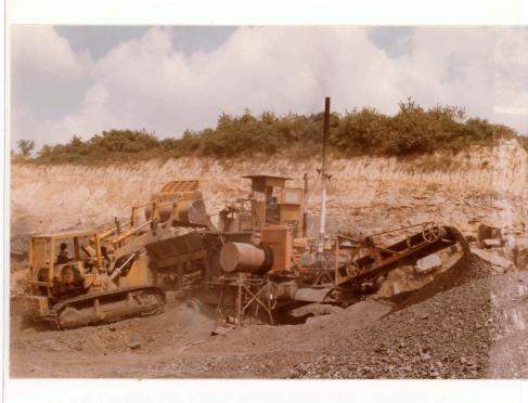
Operations in the pit. After being blasted, the rock is loaded directly into crushing machine loacted in the pit. Stone is used for road ballast a and general construction.
