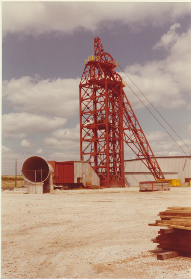
Headframe for man-and-materials shaft, and fan, at main portal of Crown III Mine.
