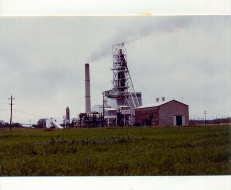
Skip shaft of the Hillsboro Mine, with smokestack of the C.I.P.S. power plant behind. Note twin rotary crushers (just below stack) and overland conveyor belt that carries crushed coal from the mine to the power plant.
