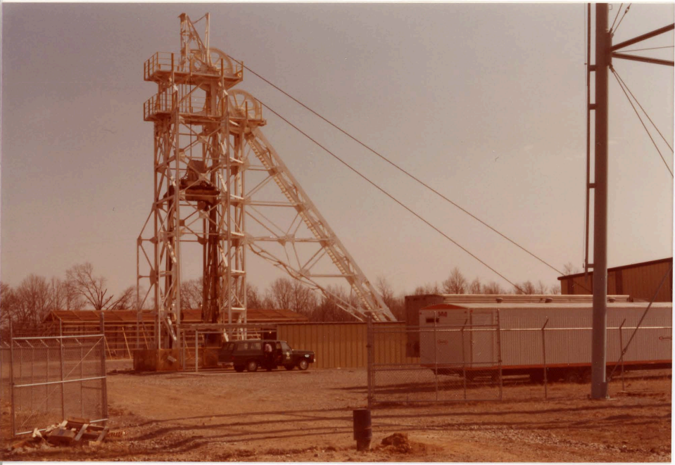
Headframe at No. 3 Portal, Orient No. 4.
