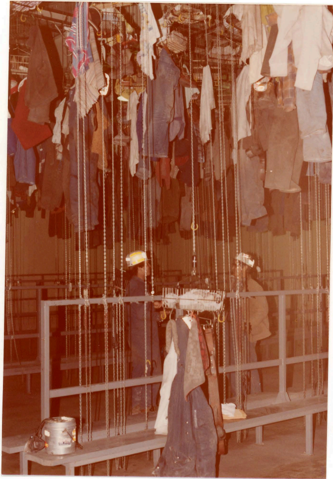
Change room, No. 3 Portal
