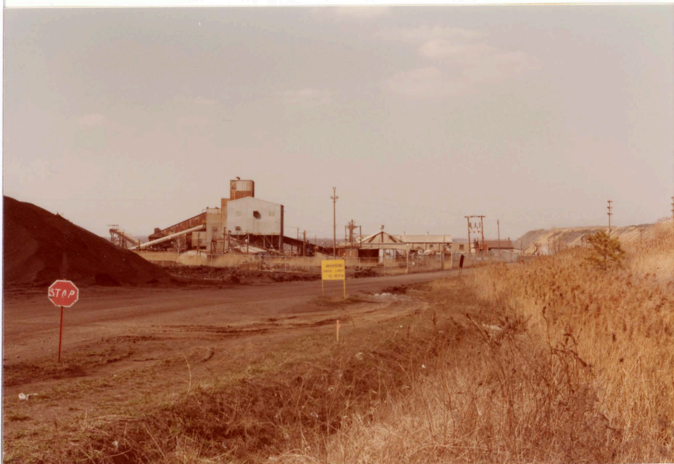
Preparation plant at old portal of Orient No. 4 Mine, looking north. Photo by John Nelson, March 24, 1981.
