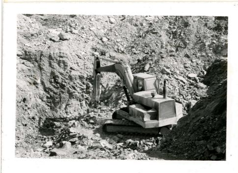
This John Deere 690-B excavator is the only piece of earth moving equipment in the mine. The top of the coal seam is just being uncovered.
