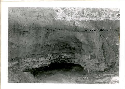
Partially caved abandoned underground mine opening in southwest part of old pit. In lower part of photo (ruler) are Energy and Anna Shales (weathered to light color and blocky appearance. Above the Anna Shale is some 12 feet of unconsolidated Pennsylvanain clay, silt, and sand, with stringers of coal. It is an unusual type of channel-fill deposit, from what I can see.
