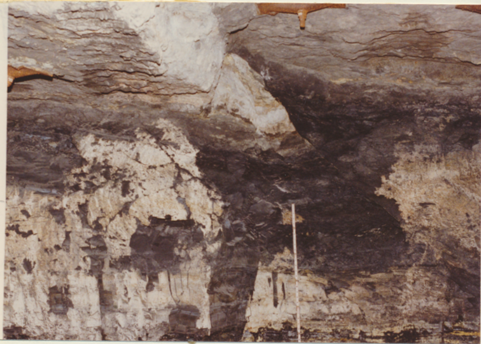
Loc. 5, 4th North Panel off Main West (east rib of No. 1 entry). North branch of Crown Fault appears as a reverse fault, with Anna Shale on south (right) thrust up and over thin Brereton Limestone and Anvil Rock Sandstone on the north.
