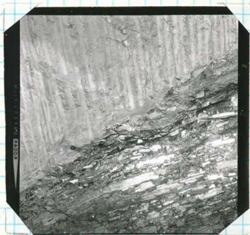
Looking into northeast wall of 45° cross-cut. Shows close-up of margin of cut-out. Note small "barbs" of coal extending into siltstone. Knife at right center for scale.
