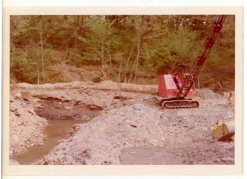
Malone Mine stripping operation. Coal seam is visible at back of water-filled pit.
