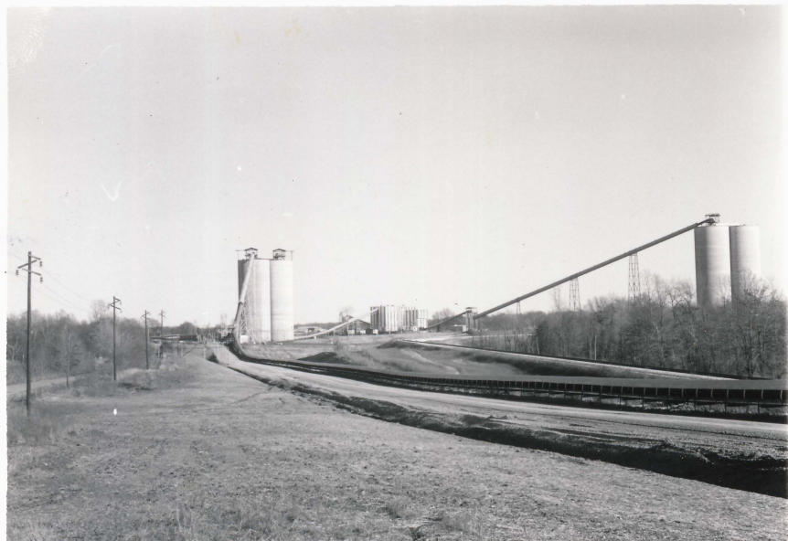
East North facing view of the raw coal silos, overland conveyor, prep plant, and clean coal silos at the Old Ben 27 Mine. Overland conveyor brings coal from O.B.25. JTBpp 11/17/77
