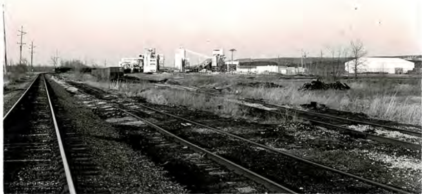
Dilapidated tippel of the Spartan Mine, Zeigler Coal Company. In the distance can be seen a coal-storage silo at the new central cleaning plant that serves both the Spartan Mine and Mine No. 11. Photo by John Nelson, March 1981.
