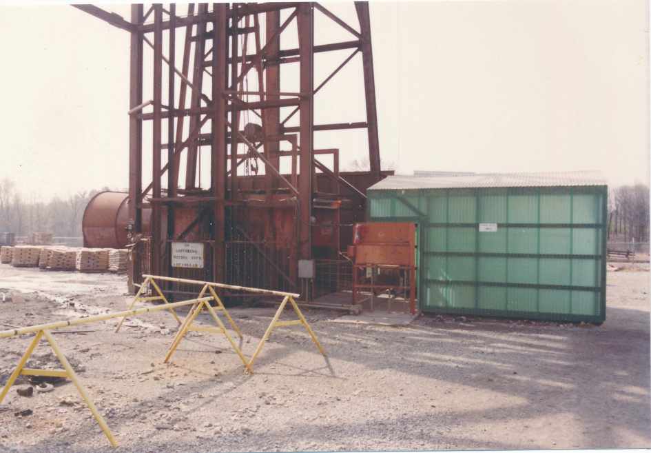
Man-and-materials shaft at Old Ben Mine No. 27
